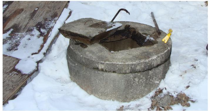
*It is important to regularly inspect and maintain your well and test the water. This is a drilled well located in a pit (these are no longer allowed to be constructed). If you have a well located in a pit, you could upgrade it so that the well casing extends at least 40 cm above the ground. NEVER ENTER A PIT.*
