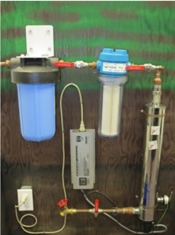
*An example of a filter and ultraviolet disinfection system.*
