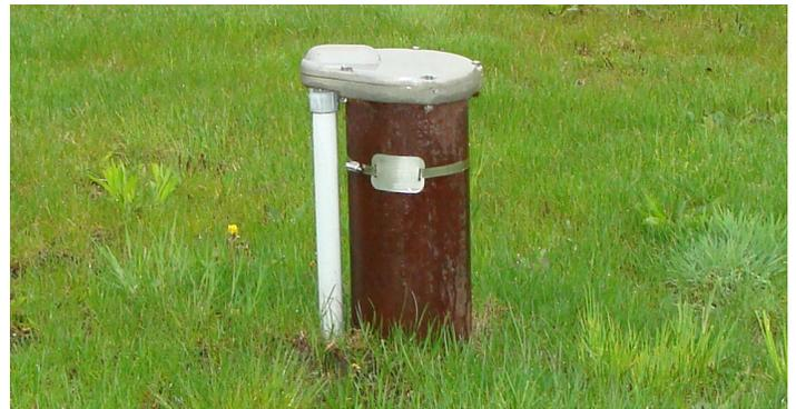
*Properly constructed drilled well shown with a vented and vermin proof well cap, electrical conduit for submerged pump (to left of well casing), identification tag (linked to Water Well Record), casing extends at least 40 cm above the ground, and ground that is mounded away from well casing.*
