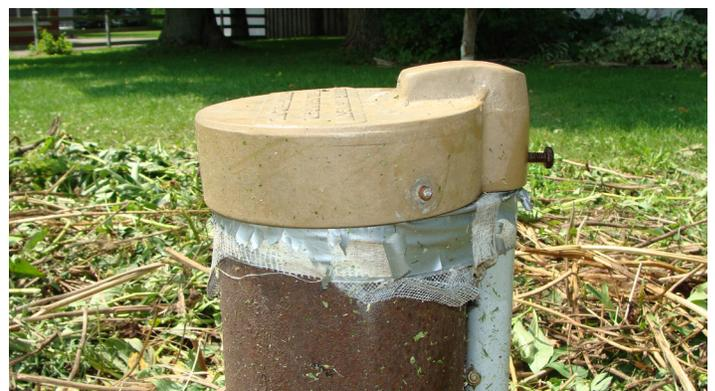
*An inadequate well cap may allow pests and other types of contamination to enter into the well, and may not allow for proper ventilation.*
