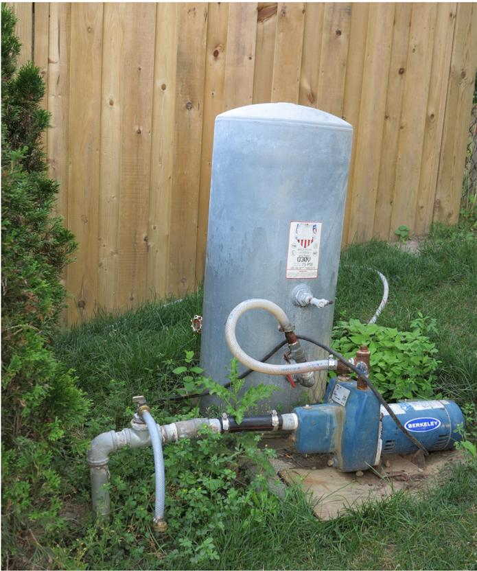
*A well point (sand point) with a pump and pressure tank on the ground. These types of wells work in areas where the water table is high as they are not very deep. They are susceptible to surface contamination and changes in water table level. This well is used during the warmer months and winterized for colder months. Plumbing can also be installed below the frost line for year round use.*
