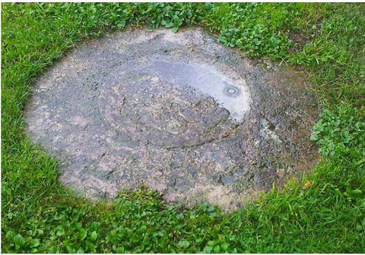
A dug well. The well cap is located close to the ground and the well is prone to contamination. Know where your well is, how it is constructed and maintained, and how vulnerable it is to contamination.
